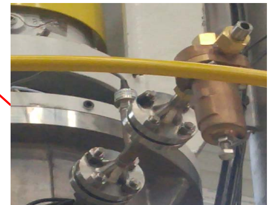
[Safety V/V] Pre. Buffer Zone (4.5bar)
