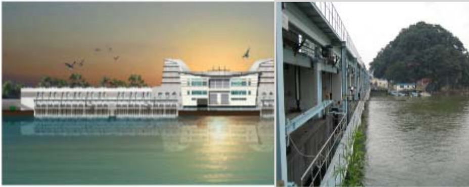
Noksan Drainage Pumping Station
