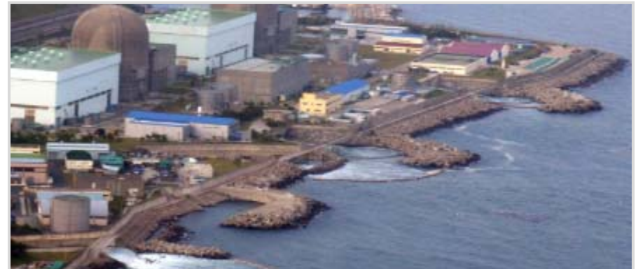
Intake Pumping station for Circulating water system of Kori Nuclear Power Plant 3&4
